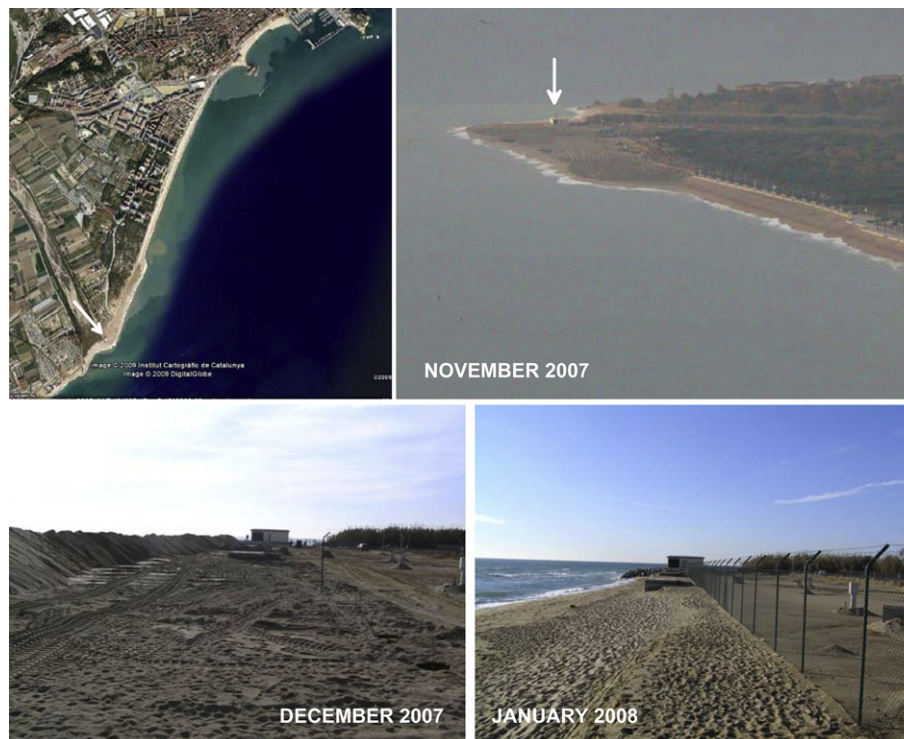
Fig. 8. Emergency beach nourishment at South s'Abanell beach during at December 2007. Top left by courtesy of Google Earth. The arrow in top photos indicates the relative position of station with respect to the shoreline just after the works. Bottom: beach just after the works (left) and one month later (right).
