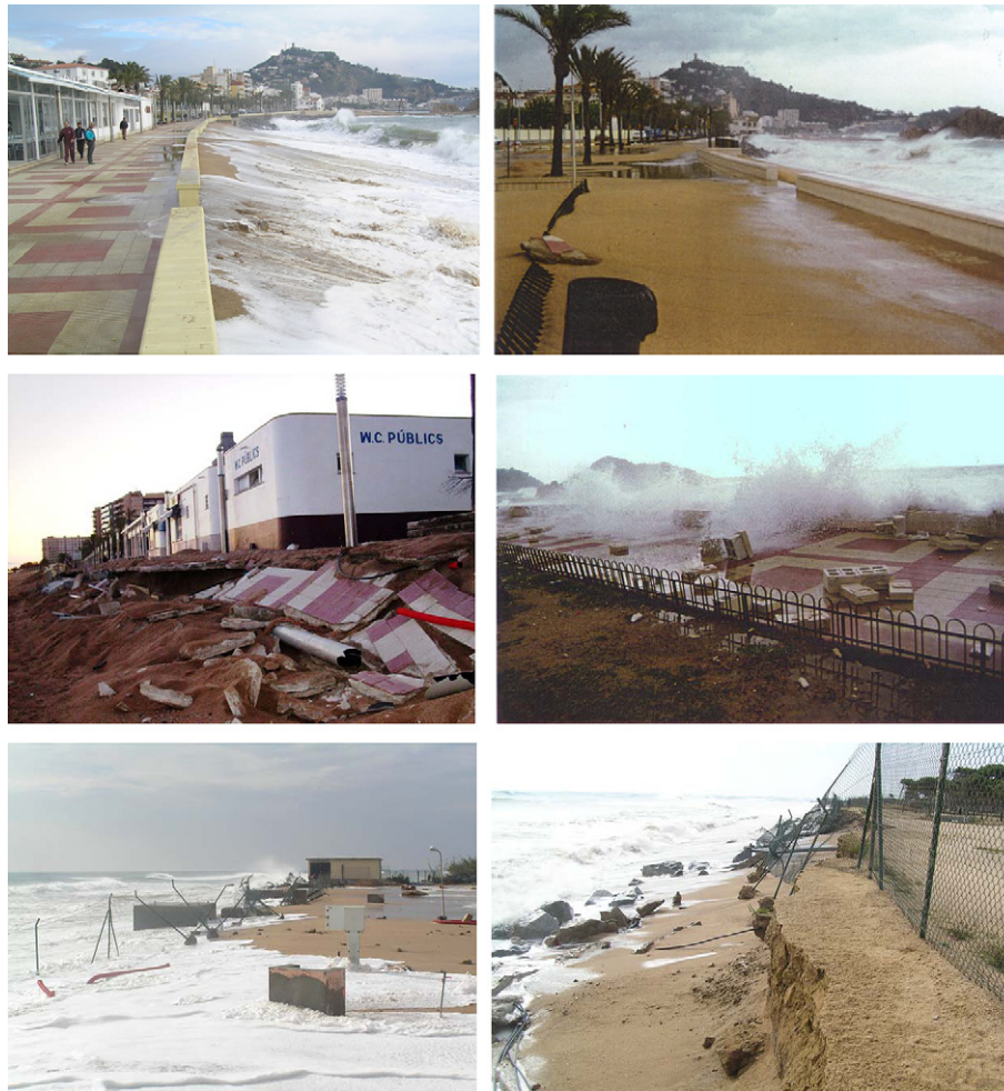
Fig. 5. Coastal protection problems in s'Abanell beach. Top: minor problems due to beach and promenade overtopping. Middle: severe problems affecting promenade stability. Bottom: severe problems affecting infrastructures of a desalination plant and the limit of campsites at the S part of the beach.
