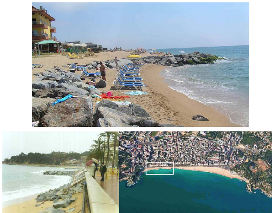
Fig. 7. Recreation malfunctions due to large erosion of the subaerial beach (top) and due to affectation of beach accesses and services due to extreme shoreline re-orientation (bottom).
